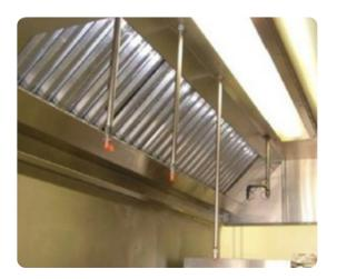
However, too much ozone would result in discharge of ozone from the exhaust, which could be harmful to human health. Whilst the World Health Organisation sets a long term ozone exposure limit of <0.05ppm, Geoff says Exoair sets its own maximum ozone discharge limit at just 0.04ppm, (that's 40 parts per billion).
