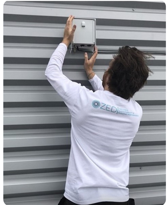
ZED used Aeroqual AQY 1 Micro Air Quality Monitors to conduct real-time air quality analysis of busy shopping centers.
